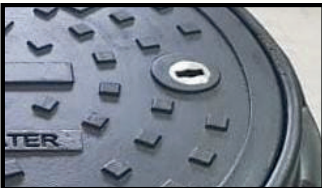
Condition of the socket type keyhole lifting arrangement of JK FRP manhole covers.
