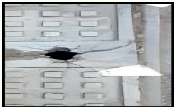
Condition of the Regular keyhole lifting arrangement of other make FRP manhole covers.
